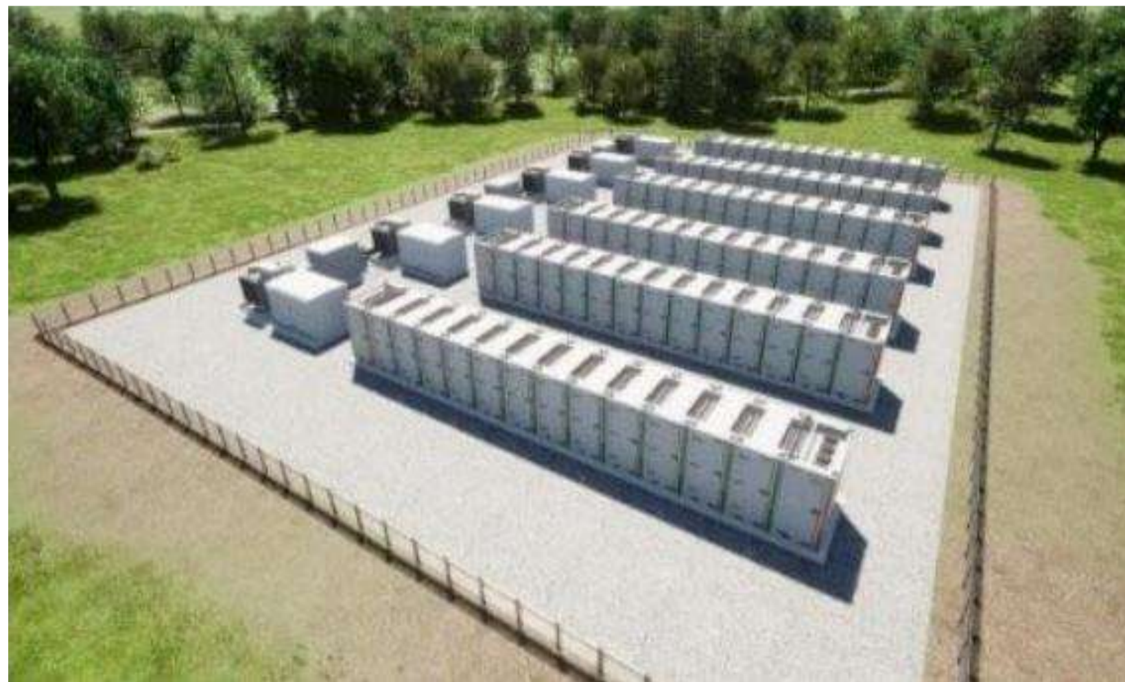
Typical Battery Energy Storage System (BESS)
