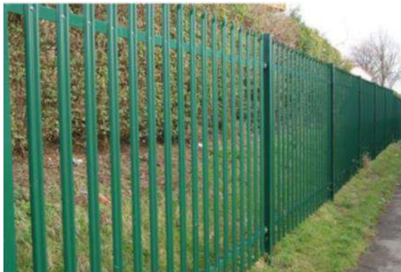
Figure 3 Example image of palisade fencing
